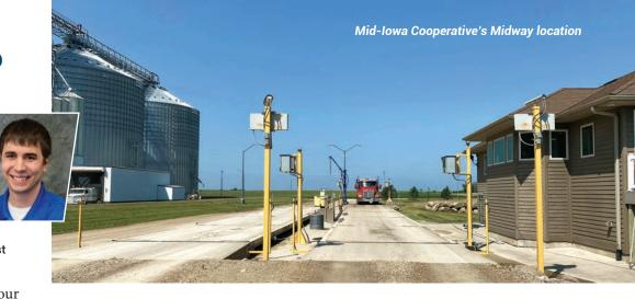
data on the screen, which helps reduce errors. When you pull onto the inbound scale, the system will also record the inbound weight.
